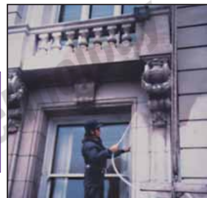
Figure 6. Spray application of silanes on large structures.
